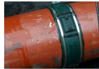
Permanently Installed Monitoring Systems (PIMS)
