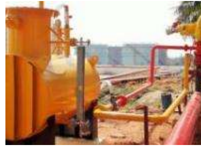
Foam System @ HPCL Karnataka
