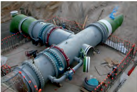
WATER TREATMENT PLANT
