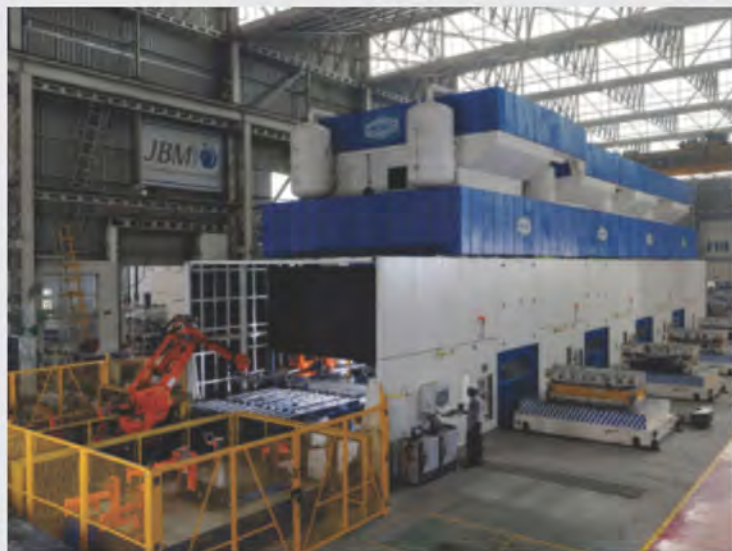
<<< 12-8-8 Automated Tandem Press Line with sound/dust proof enclosure supplied to JBM Group at their plant in India. The Press Line is equipped with Robotic Automation and is being used for producing skin component for Suzuki Maruti.
