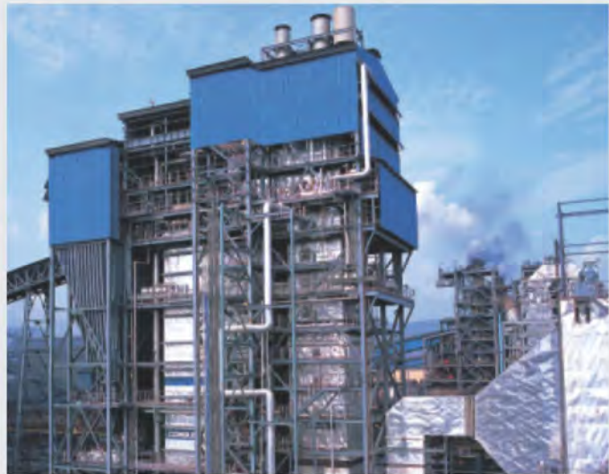
150 TPH CFBC Boiler with Compact Separator for Jindal Steel & Power, Raigarh, India.
