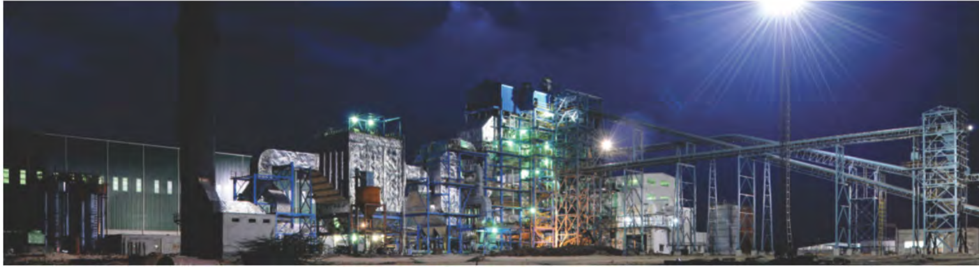
25 MW Complete Cogeneration Plant supplied on EPC basis to Coregreen Sugar & Fuels Pvt. Ltd., India.
