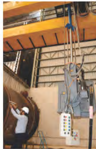
Radiography facility up to 300 mm (12") thickness using a 6MeV Linear Accelerator. We have 9 radiography halls and take more than 300,000 radiographs annually. We also have facility for X-Ray and Iridium Radiography.
