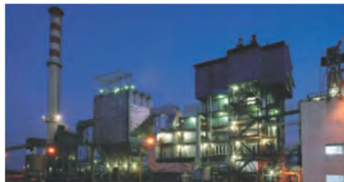
90 TPH, 67 Kg/sq.cm., 485 Deg. C Coal Fired AFBC Boiler for Gujarat Fluorochemicals Ltd. India.
