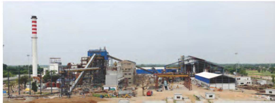
20 MW Complete Cogeneration Plant supplied on EPC basis, including Water Intake system, to HPCL Biofuels Ltd., Lauriya, India.
