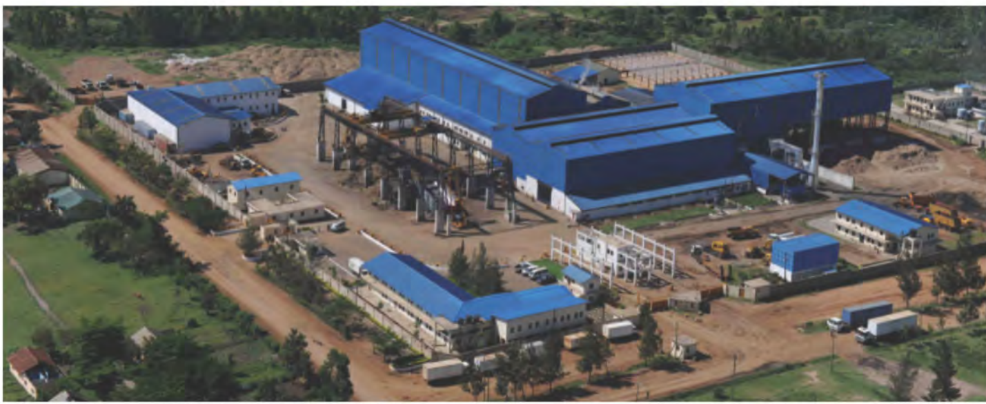
Sugar Plant set up on a turnkey basis for Kibos Sugar & Allied Industries Ltd., Kenya having a crushing capacity of 400,000 Tonnes of Cane per annum. Currently being expanded to a crushing capacity of 650,000 Tonnes of Cane per annum with Cogeneration of 110,000 MW per annum.
