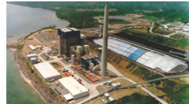
486 MWe PC Fired Boilers for Queson, Philippines commissioned by Foster Wheeler.
