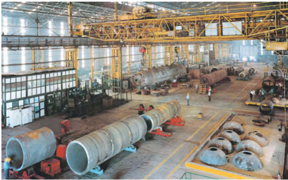
One of the 7 Pressure Vessel Bays. We also have 14 Bays for the manufacture of Boiler Pressure Parts.
