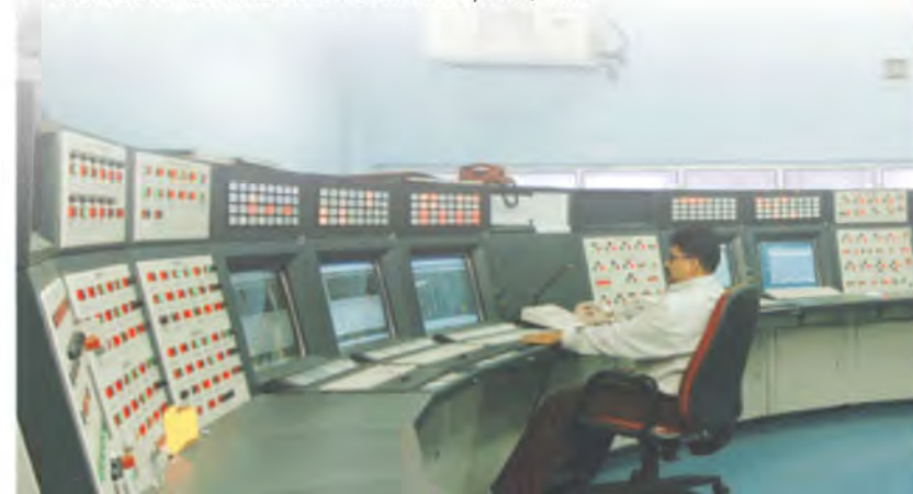
Boiler Control Room at Chennai Petroleum Corp. Ltd., India.
