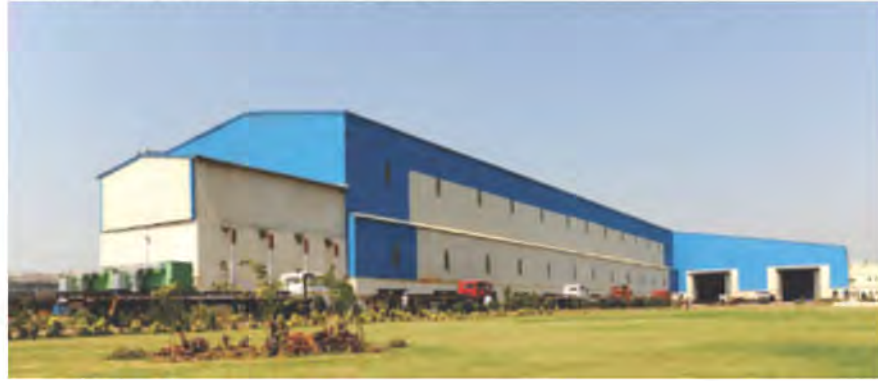
Isgec Plant at the port town of Dahej (Gujarat), India. The shop has been set up especially for the manufacture of large and heavy equipment for the overseas market.
