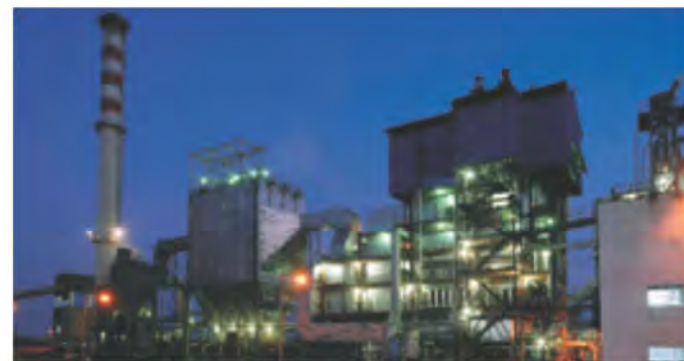
90 TPH, 67 Kg/sq.cm., 485 Deg. C Coal Fired AFBC Boiler for Gujarat Flourochemicals Ltd. India.
