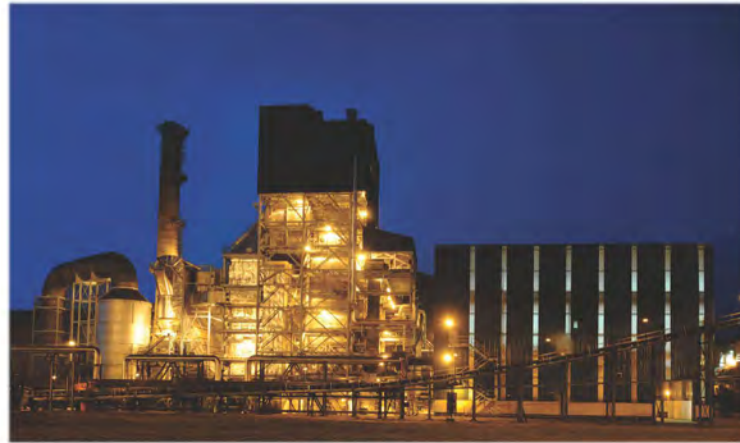
30.4 MW Complete Cogeneration Plant supplied on EPC basis to Zambia Sugar Plc. (a subsidiary of Illovo Group of South Africa) Nakambala, Zambia.
