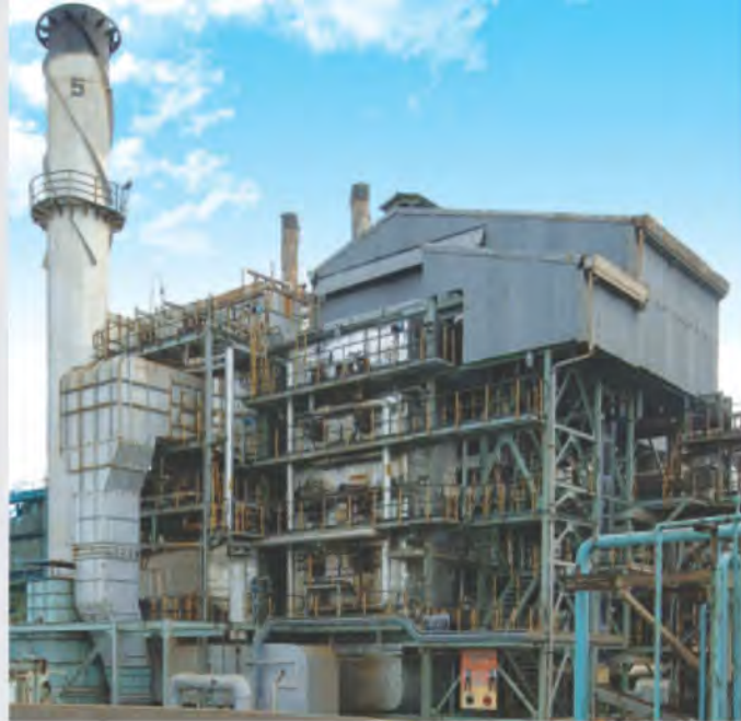
<<< 100 TPH, 50 Kg/sq.cm.g, 430 Deg. C, HFO / Natural Gas fired Boiler supplied to Chennai Petroleum Corporation Ltd. Chennai, India.
