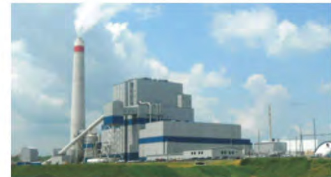
World's largest Super-Critical PC Fired Boiler (770 MWe) using Benson Vertical Tube Evaporator design commissioned by Foster Wheeler at Longview Power LCC, USA.
