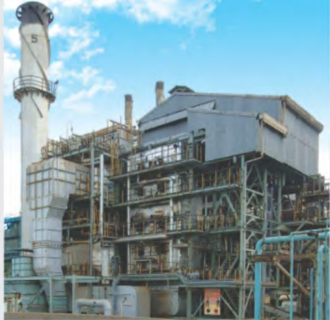
<<< 100 TPH, 50 Kg/sq.cm.g, 430 Deg. C, HFO / Natural Gas fired Boiler supplied to Chennai Petroleum Corporation Ltd. Chennai, India.
