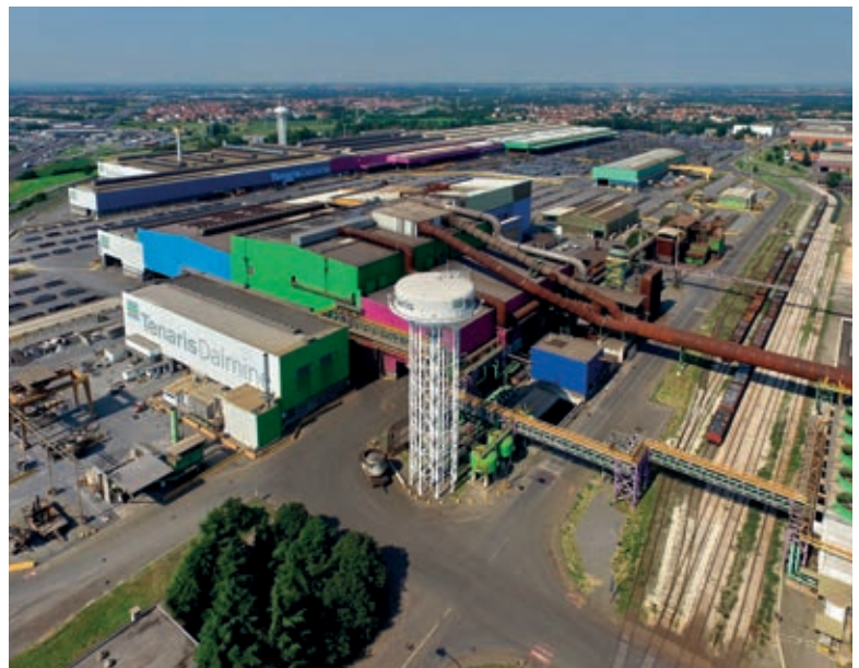
TENARISDALMINE'S STEEL SHOP AERIAL VIEW
