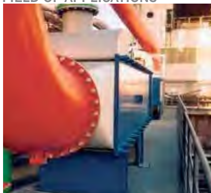
Low pressure vapour condenser
