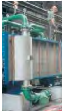
Liquid/liquid energy recovery
