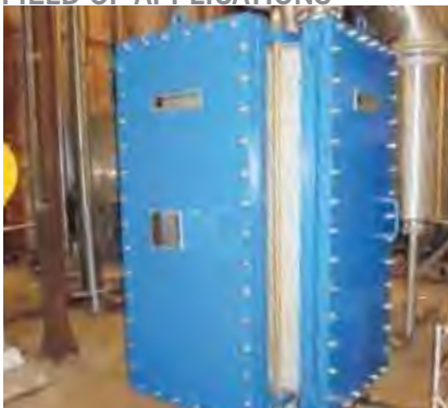
Platulaire® type X 4 doors on distillery vinasses
