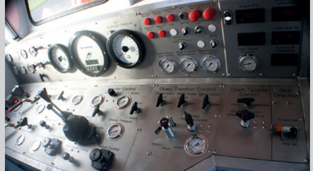
CTU Control Panel
