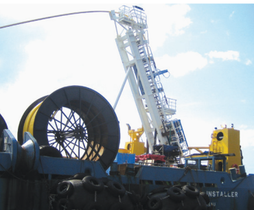
Coiled line pipe J-Laid from adjustable tower.
