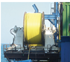
Coiled line pipe S-Laid from a DP vessel (left), and Coiled Line Pipe laid as piggy back from a DL barge. (right)
